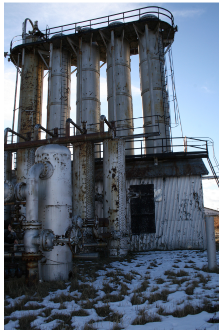
Figure 1: Exterior view of the absorption building located at the Turner Valley Gas Plant. The image shows the five absorption towers, and the corrugated iron sheathing. (Parks Canada Agency.1995)
