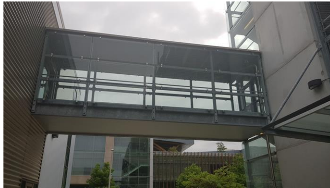
Figure 2: University of Windsor Parking Garage Bridge
