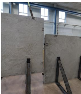
(c) Placement of second wall panel
