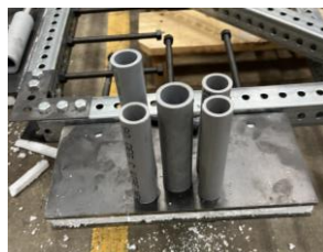
(c) Protective conduits for bolts during casting
