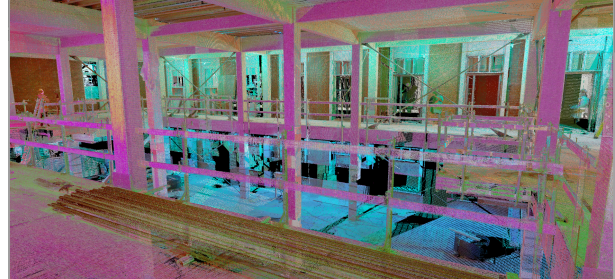
Figure 3b: Internal View on D-Level
